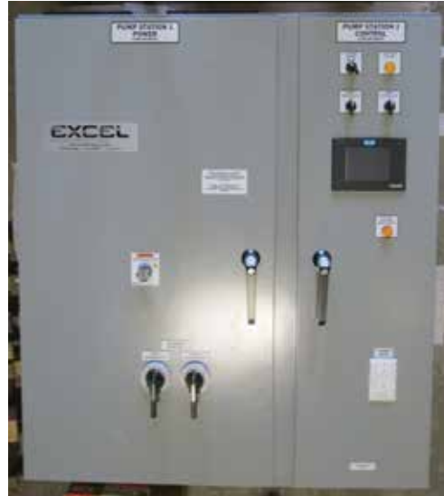
Arc-Sentry Control Panel: Design reduces arc flash hazards and includes user friendly controls
