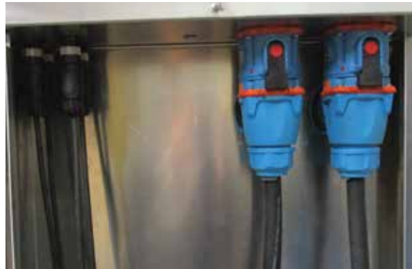
Electrical Plugs and Receptacles: Ensures correct pump rotation and reduces installation, maintenance and service time
