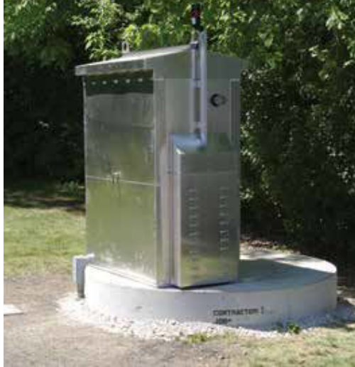
Above Ground Enclosure: Eliminates Confined Space Safety Hazards and reduces Real Estate Requirements
